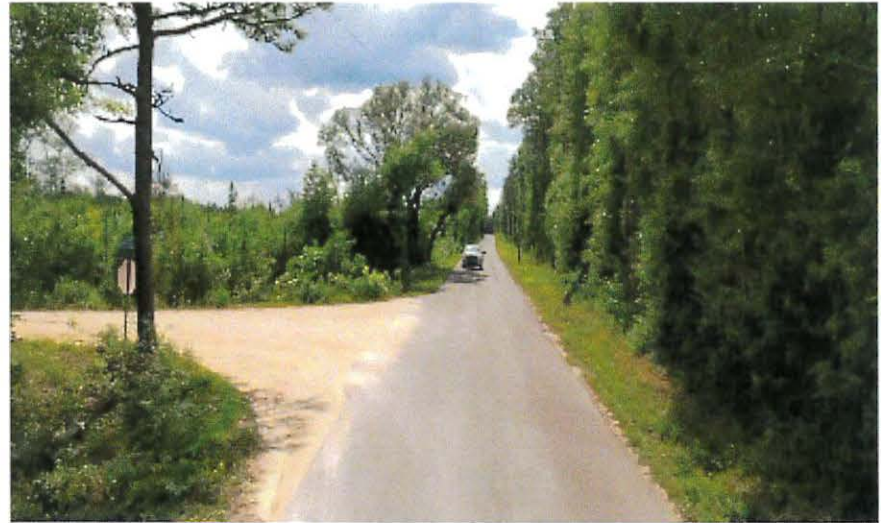
Current Road Condition with Hot-Mix Asphalt.
